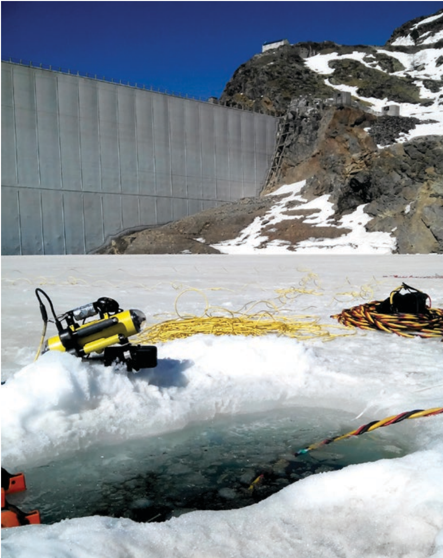
Mini-ROV Guardian equipped with a Blueview sonar, ready to operate on dam
